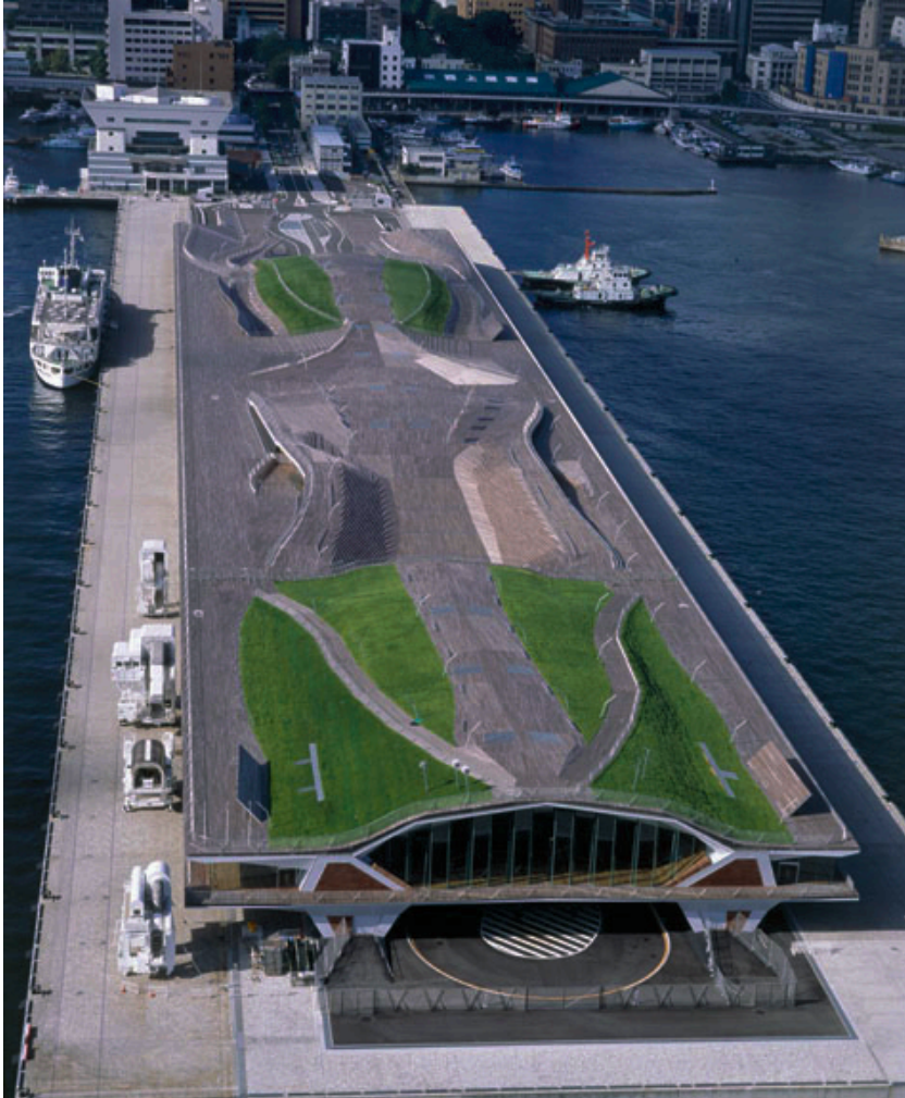
Figure 3. Yokohama International Passenger Terminal, 2002, FOA Architects; photo taken by Satoru Mishima. https://commons.wikimedia.org/wiki/File:Osanbashi_Passenger_Terminal_-_Satoru_Mishima.jpg . CC BY 3.0.
