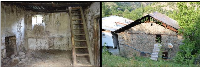
Figure 7. Wooden staircase and attic floor.
