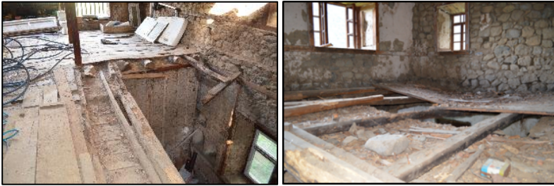
Figure 10. Roof and mezzanine flooring, respectively
