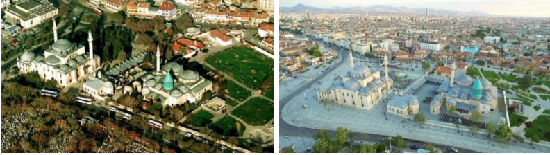
Figure 3.a. Before the Renovation of Mevlana Square and Road Widening Works and Figure 3.b. After the Renovation of Mevlana Square and Road Widening Works
