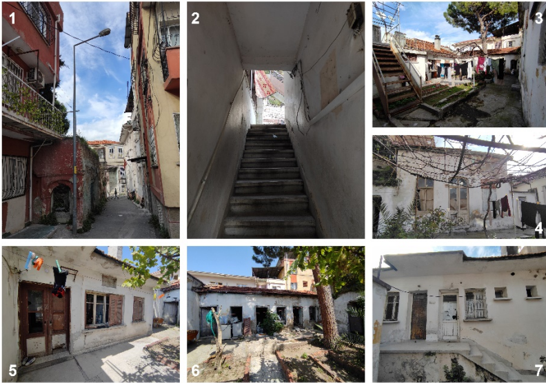
Figure 2, Views 1-7. Courtyard/Home in Pazaryeri Neighborhood. Source: (Plan) Produced within the scope of AAVS "In Other Latitudes" Visiting School (July 2023), edited by Leman Özgür; (Photos) Perin Çün's archive (2023).
